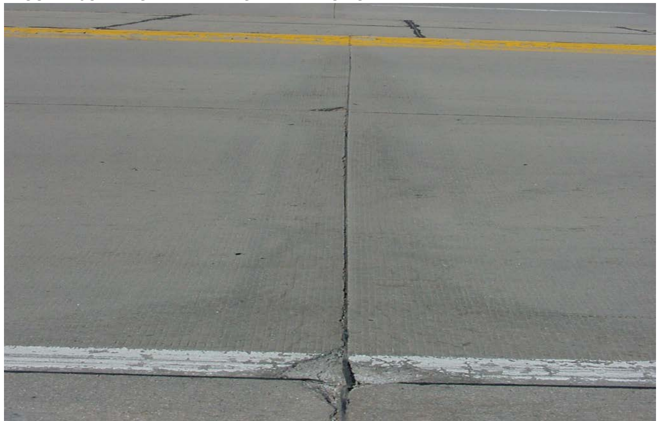
REGULAR JOINT – STAINED AND SPALLED HIGH SEVERITY
