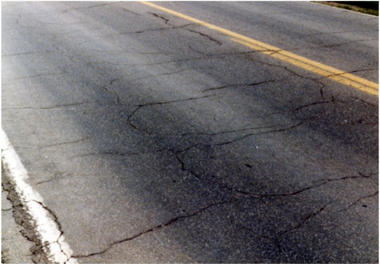
RANDOM/GRID BLOCK CRACKING – HIGH SEVERITY
