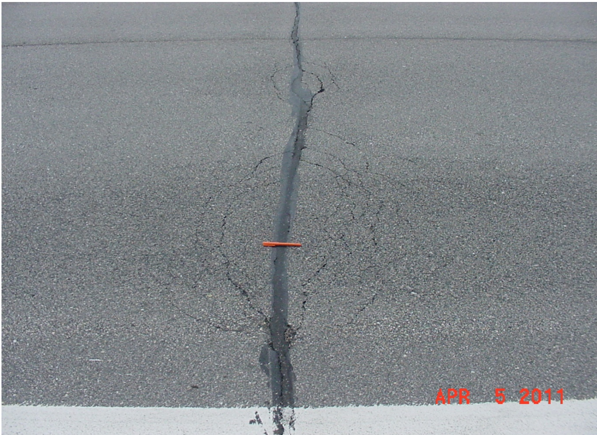
TRANSVERSE CRACKING – MODERATE SEVERITY w/ ALLIGATOR CRACKING
