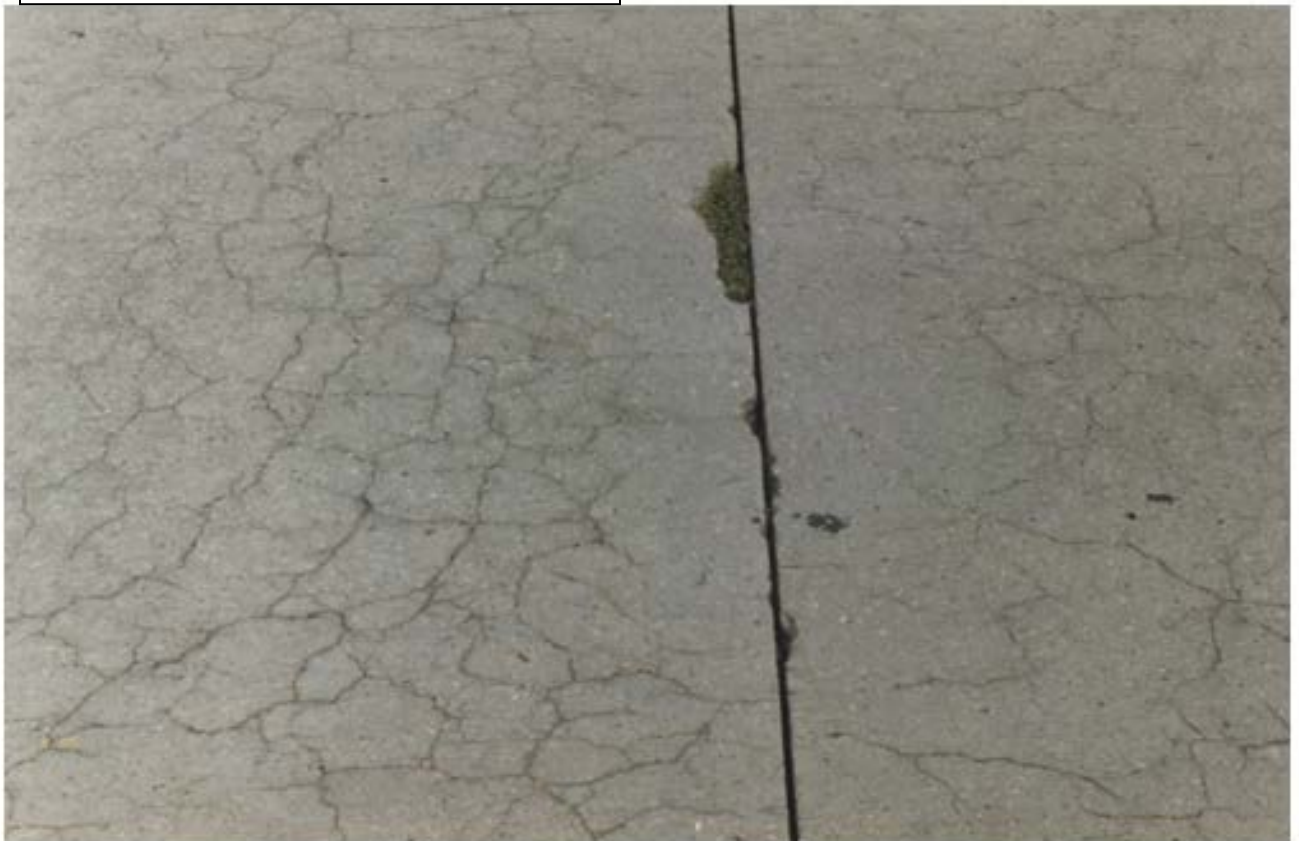
REGULAR JOINT – HIGH SEVERITY
