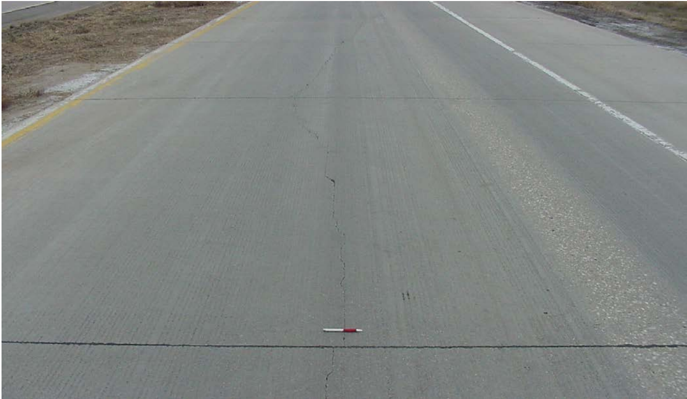
SLAB CRACKING
