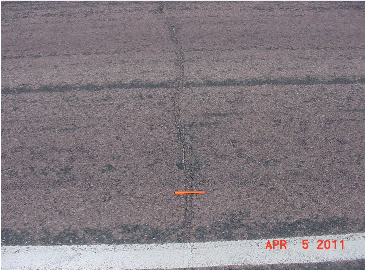
TRANSVERSE CRACKING – MODERATE SEVERITY w/ ALLIGATOR CRACKING
