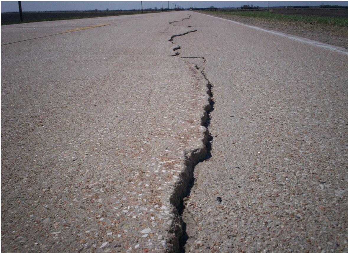
LONGITUDINAL FAULTING - HIGH SEVERITY
