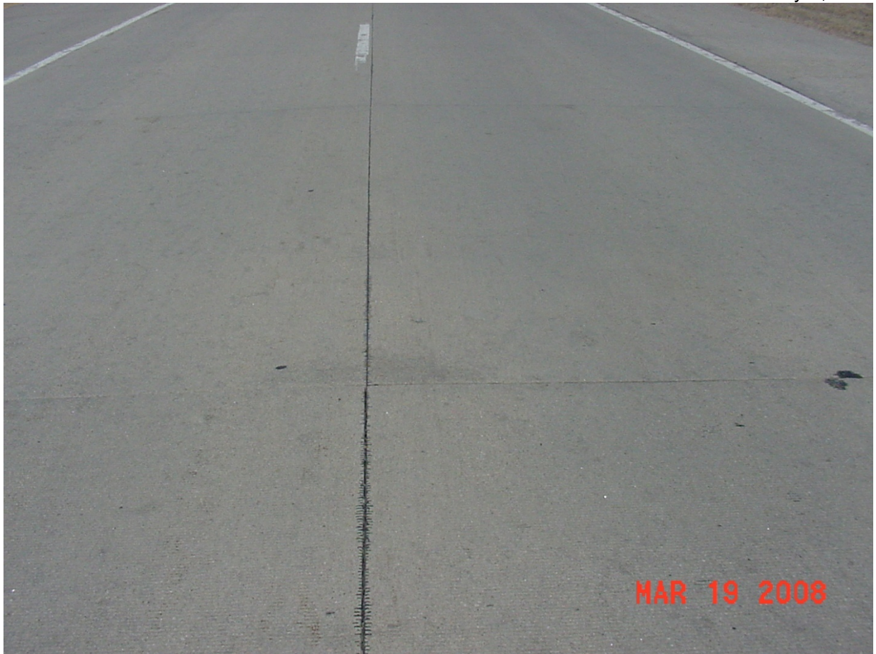
REGULAR JOINT – STAINED MODERATE SEVERITY
