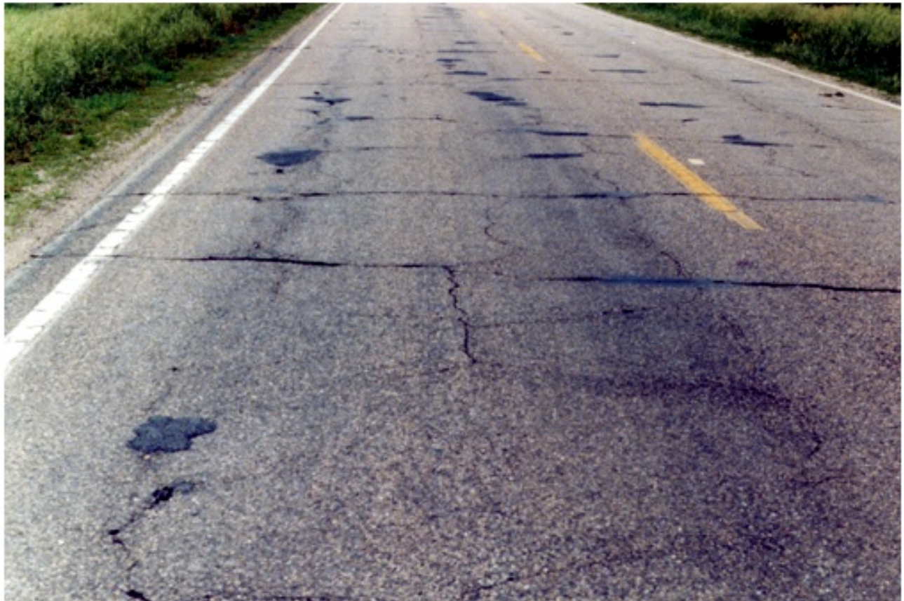
RANDOM/GRID BLOCK CRACKING – HIGH SEVERITY
