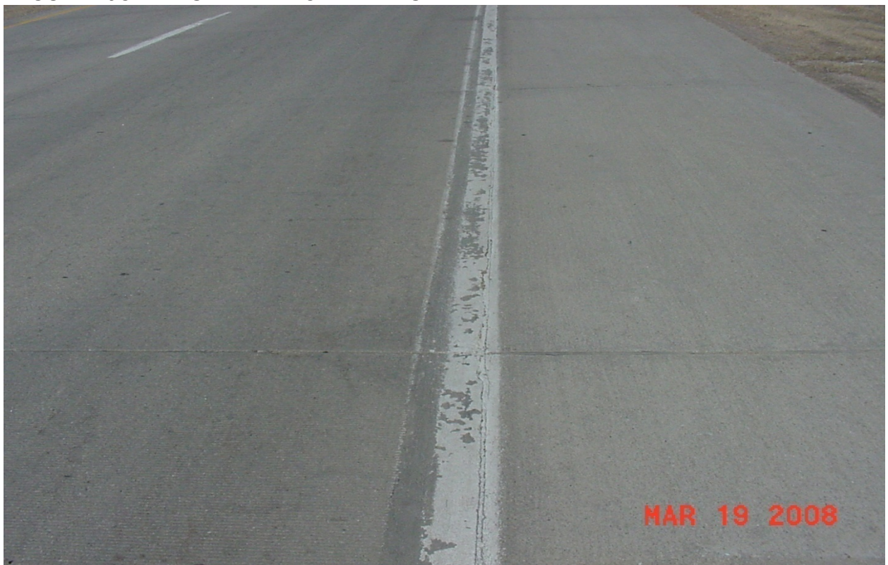
REGULAR JOINT – STAINED MODERATE SEVERITY
