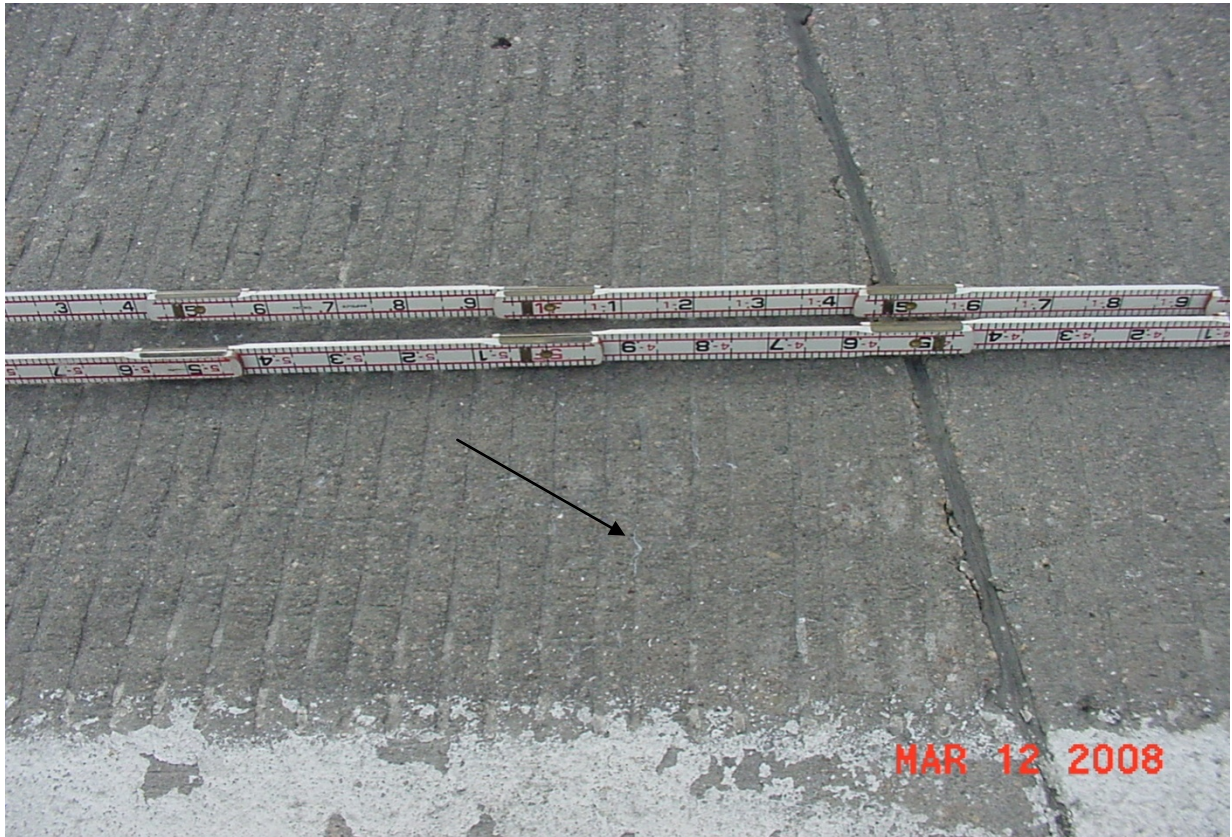
REGULAR JOINT – CRACKS SHOWING PASTE - HIGH SEVERITY
