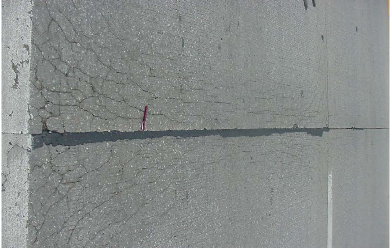
REGULAR JOINT – HIGH SEVERITY
