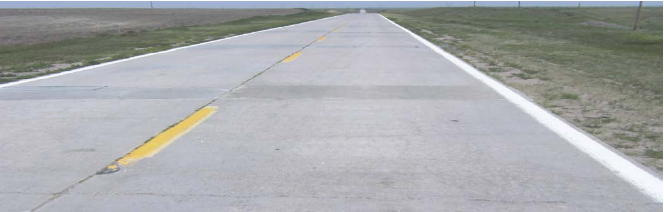
REPAIRED JOINT – MODERATE SEVERITY
