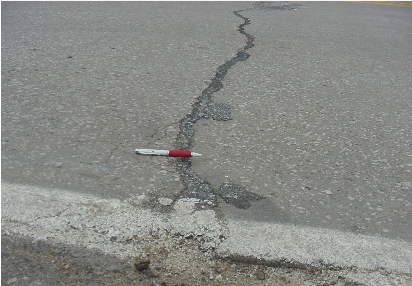
SLAB CRACKING
