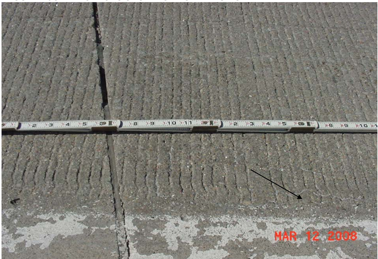
REGULAR JOINT – CRACKS SHOWING PASTE - HIGH SEVERITY
