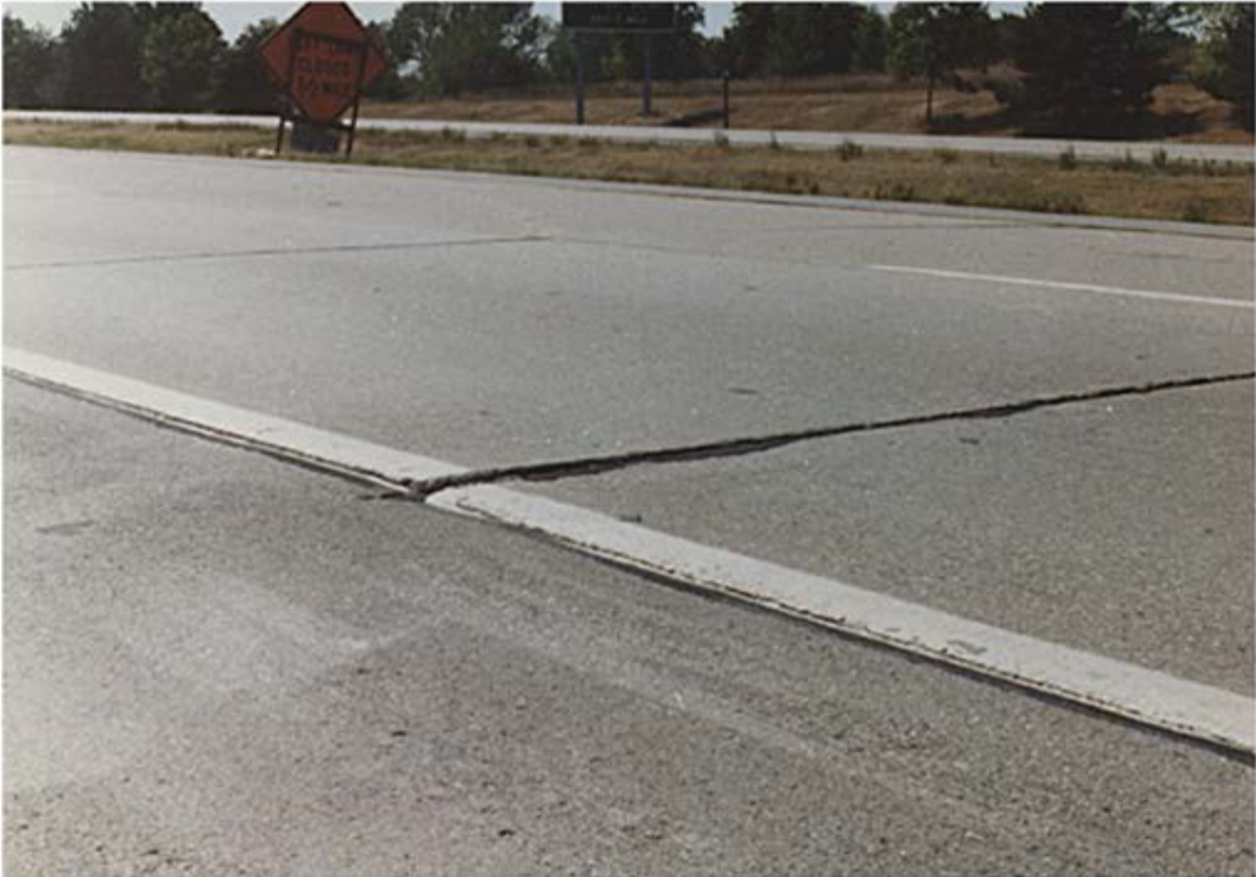
LONGITUDINAL FAULTING - HIGH SEVERITY
