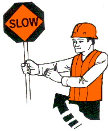
Figure 14. Releasing traffic with the slow paddle
