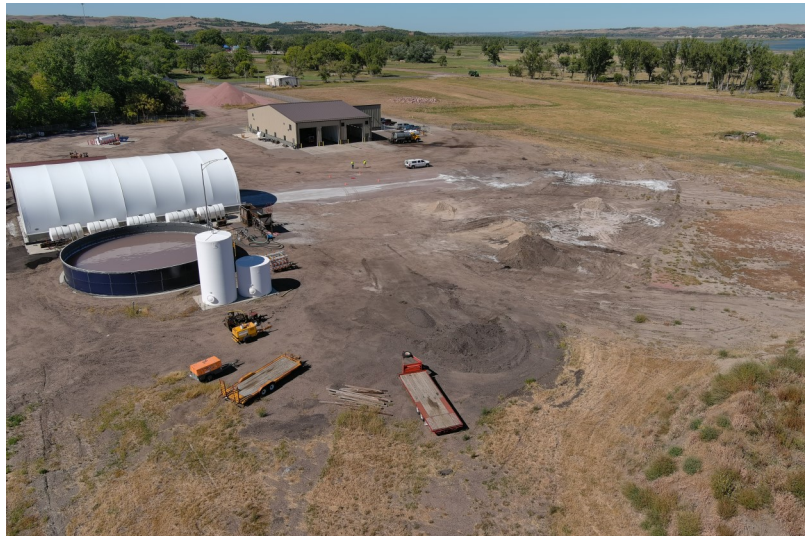
Below & to the right: NIOBRARA MAINENANCE YARD
