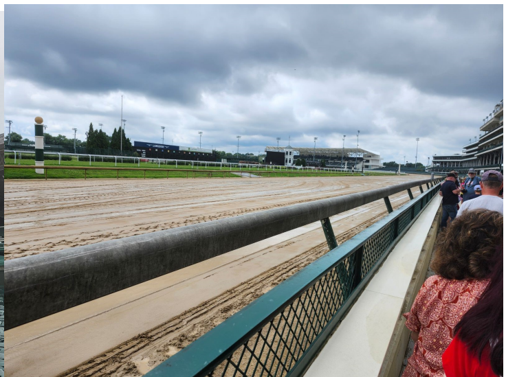
Churchill Downs. On the track they dug down 25' by hand and replaced the original soil with a mix of sand and silt with just a little cohesive material when they built this.
